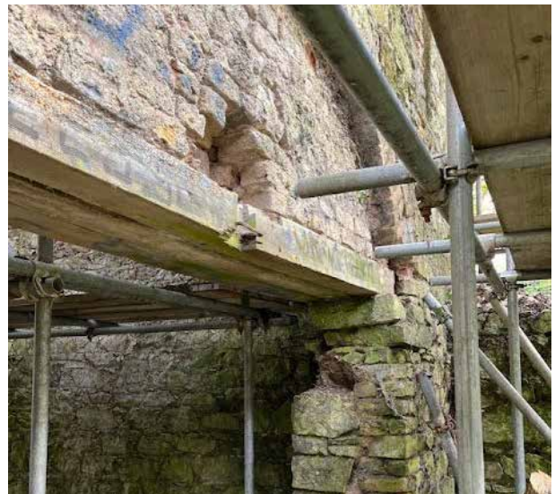
Figure 50 - Failing lintel to the opening in the south gable
