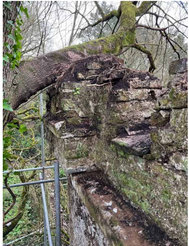
Figure 49 - Tree resting on the parapet wall
