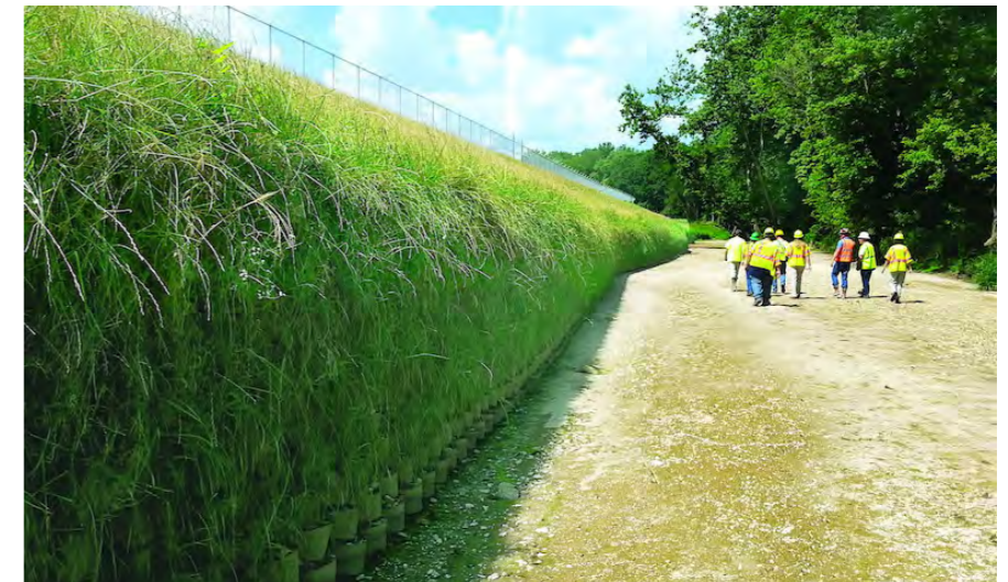
Figure 4.18: "Living" Flood Wall
