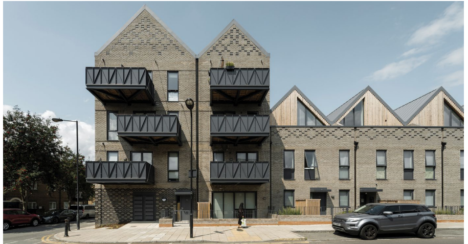
Interface to existing fine grain terrace houses- New development on the corner of King Edwards Road and Tyron Crescent
