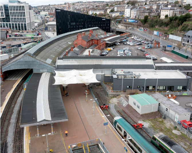
Existing Kent Station and surroundings
