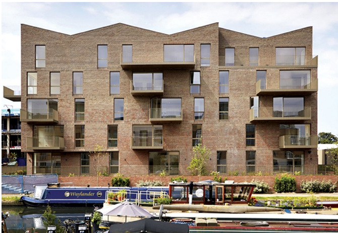
Expression of industrial character in roofscape - Brentford Lock
