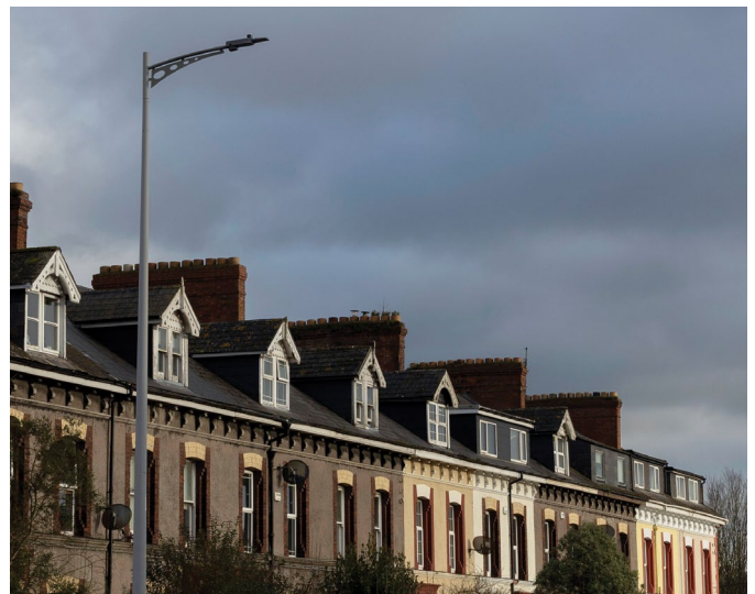
Existing houses on Victoria Road
