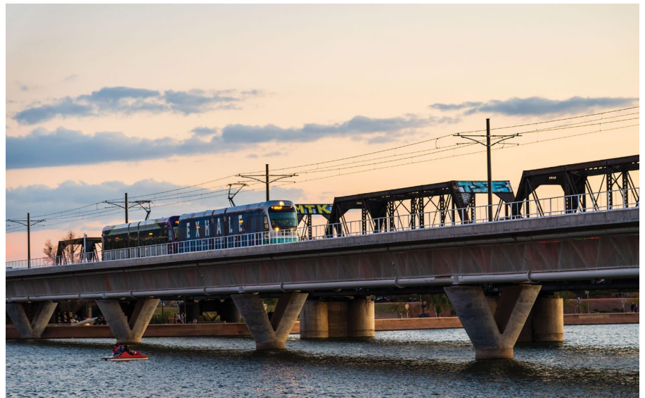
Tempe Light Rail Transit Bridge 9m width
