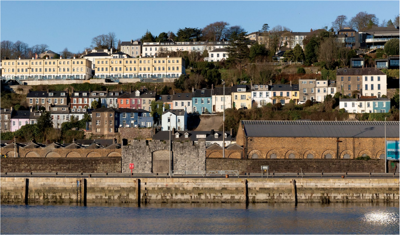
View of the historic Kent Station boundary wall
