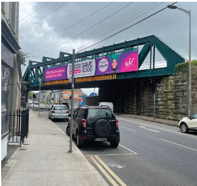
Existing Lower Glanmire Road bridge crossing
