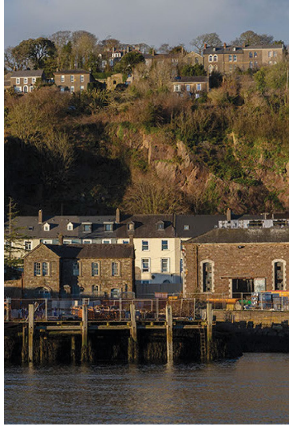
Harbour Commissioner's Workshop and slipway
