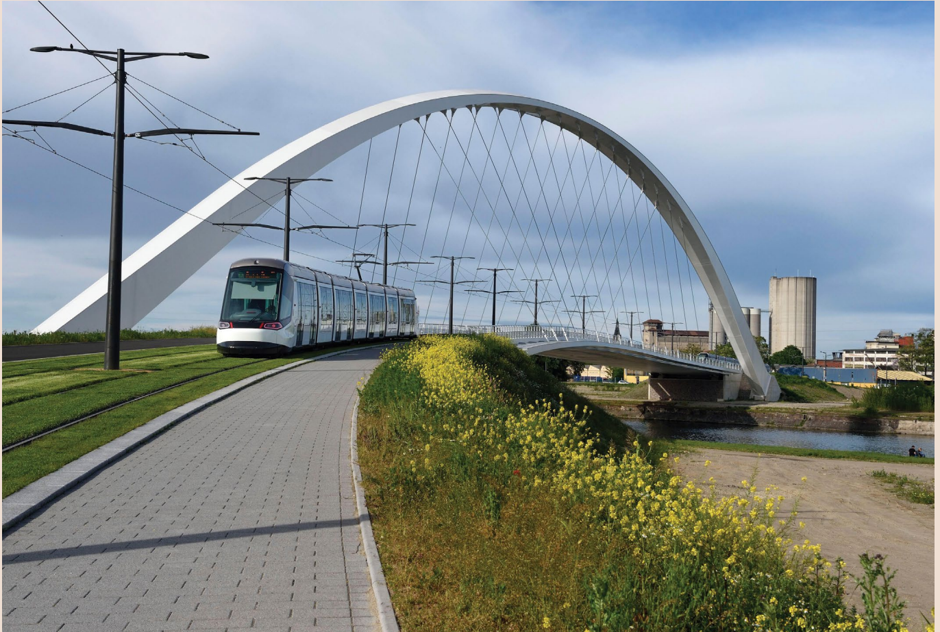
Dual track LRT, Pedestrian & cycle - André-Bord (Citadelle) Bridge Strasbourg, France
