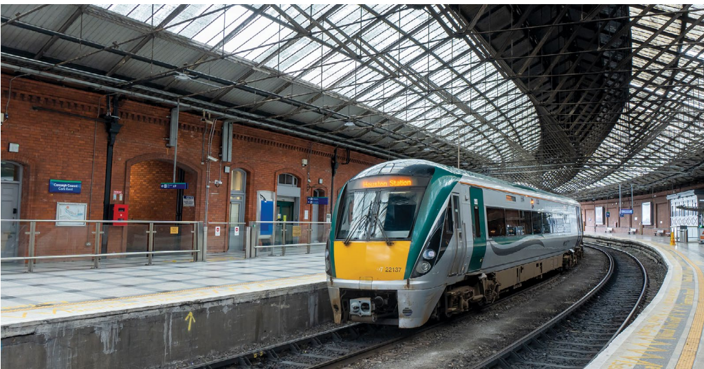
Integrated Transport Interchange at Kent Station
