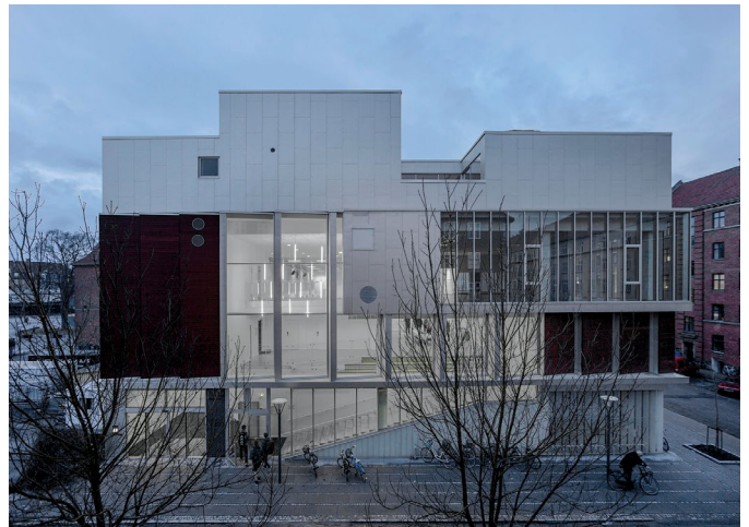
Sundbyøster Hall II supermarket on the ground floor, a sports hall on first and apartments on the top floor
