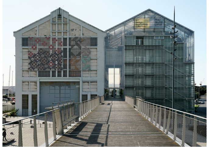
Environmental upheaval and contemporary art - FRAC Grand Large in Dunkerque's former shipyard
