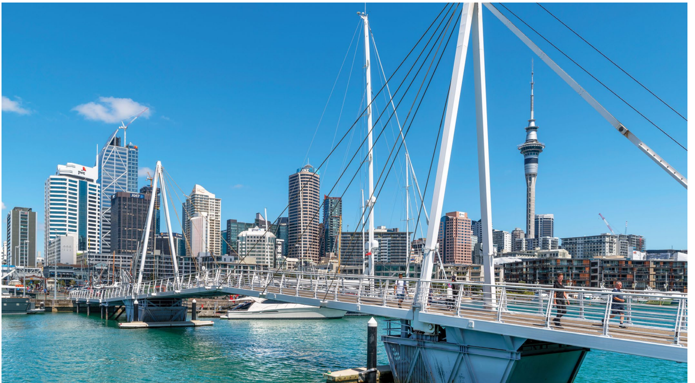
Pedestrian & bicycle - Wynard Bridge, Auckland New Zealand
