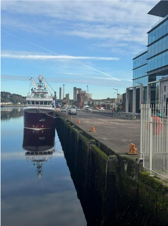
Photograph 2: Existing wharf on Albert Quay east looking downstream. The existing RC quay wall is fronted by steel sheet piles with intermittent timber fenders.
