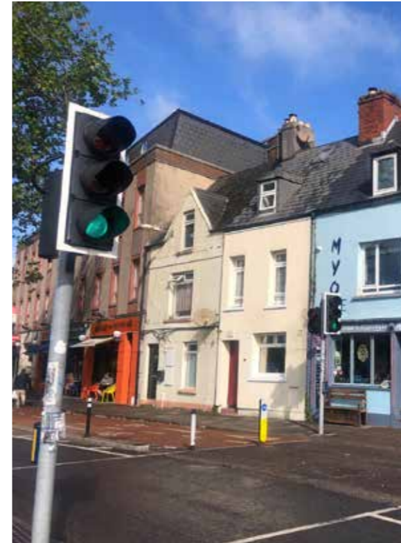
Pope's Quay: Poorly proportioned PVC windows, surface mounted utility boxes
