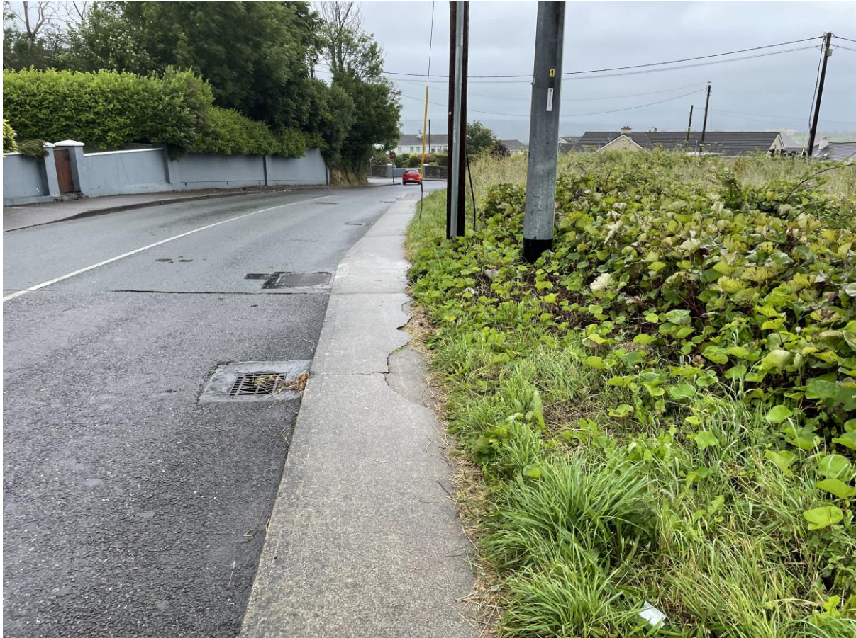
Photo A3 Utility Poles close to footpath edge and damaged footpath
