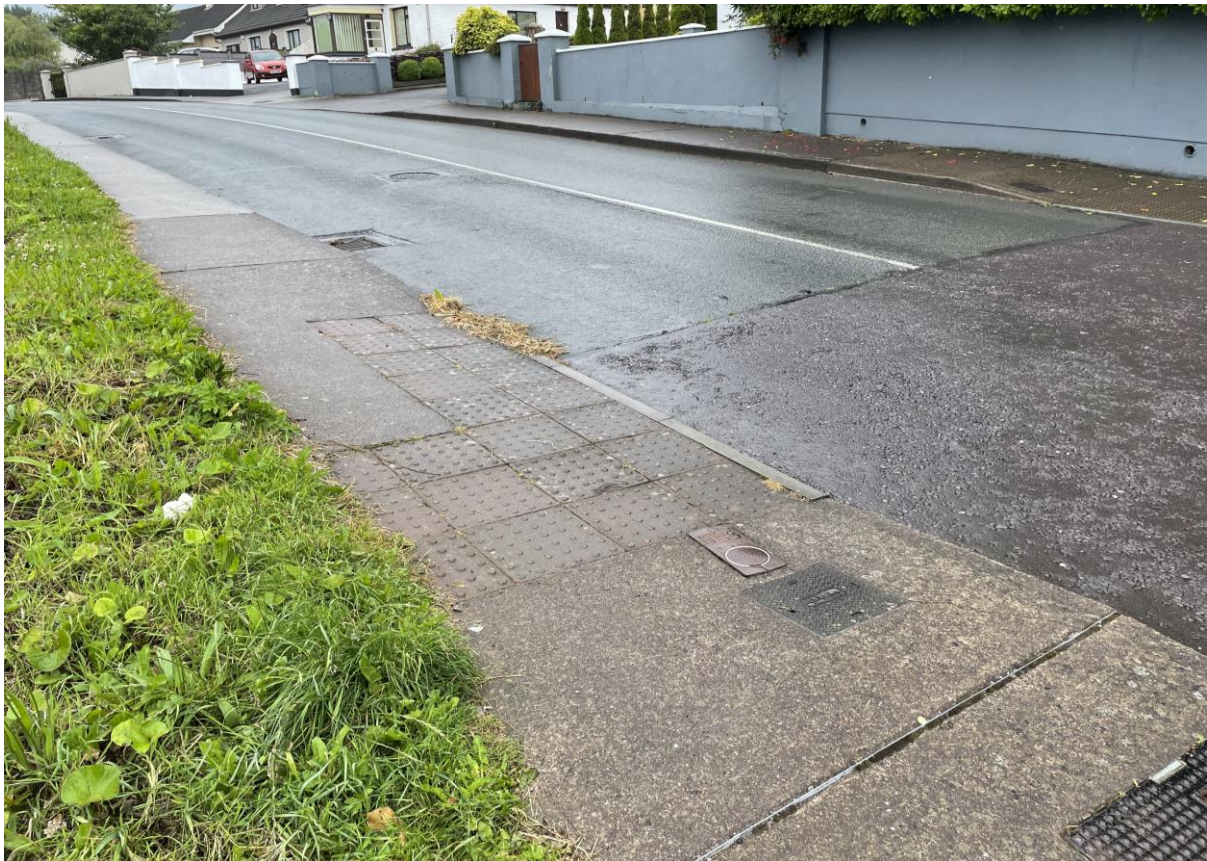
Photo A4 Existing Pedestrian Crossing on Scairt Road
