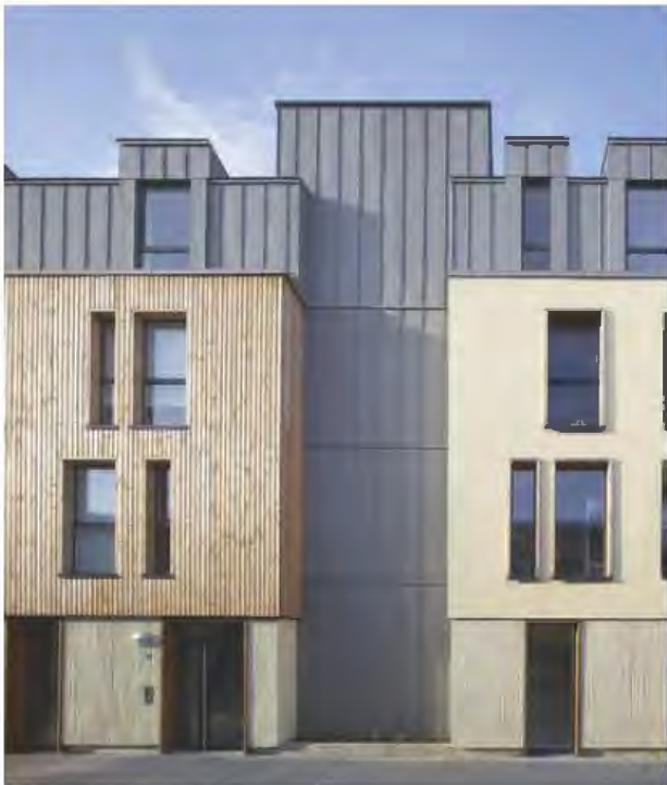
Metal cladding mixed with variety of finishes
