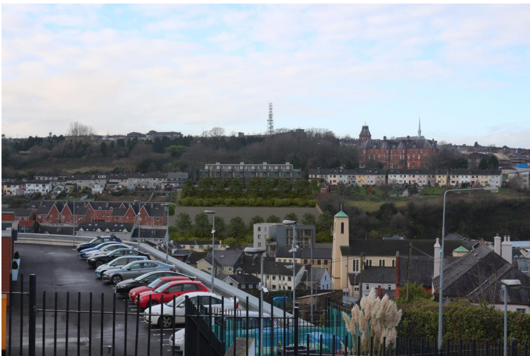
View from the Revenue Regional Office looking over to the scheme at Redemption Road.
