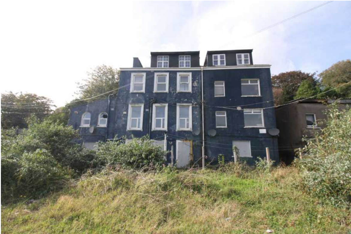
• Fig 16. Eastern view of house.
