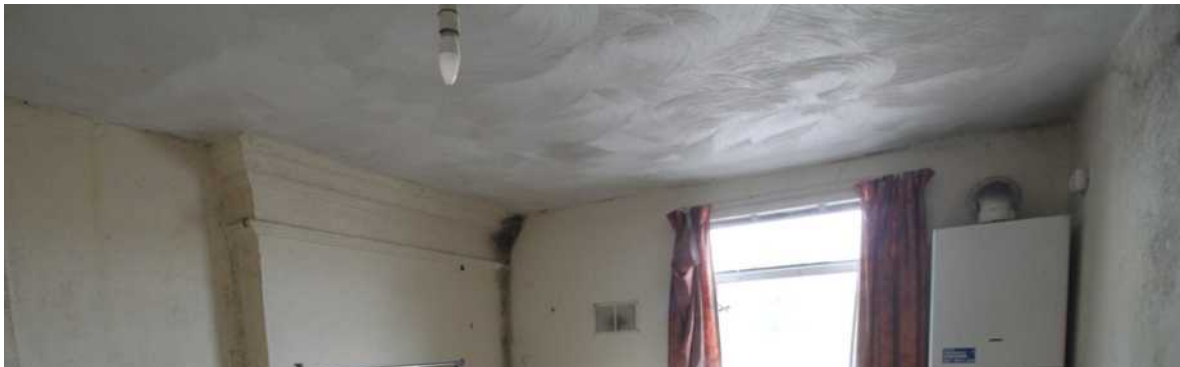
• Fig 40 & 41. Sole remaining ceiling rose and below section of an earlier cornice.
