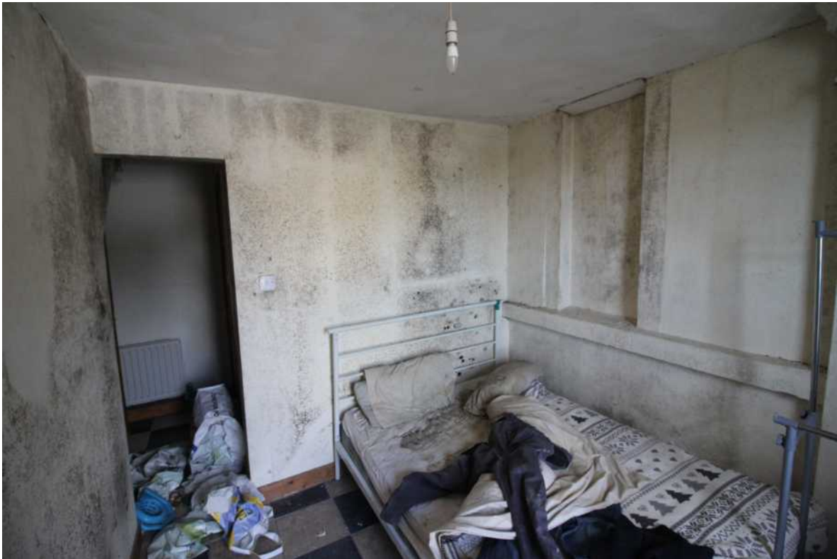
• Fig 100 & 101. Bedroom with common mould issues.
