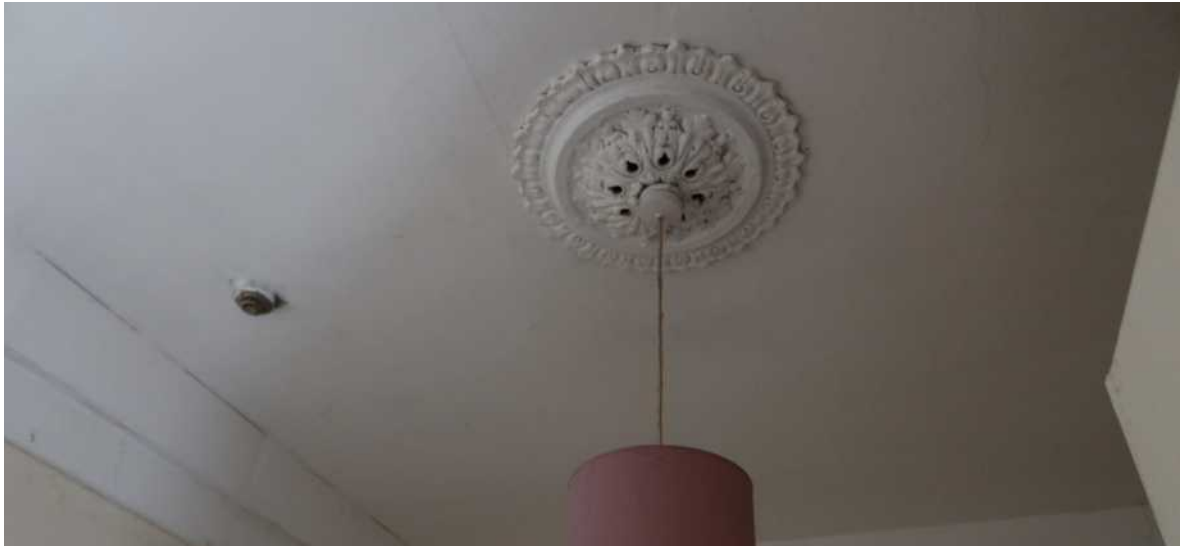
• Fig 40 & 41. Sole remaining ceiling rose and below section of an earlier cornice.
