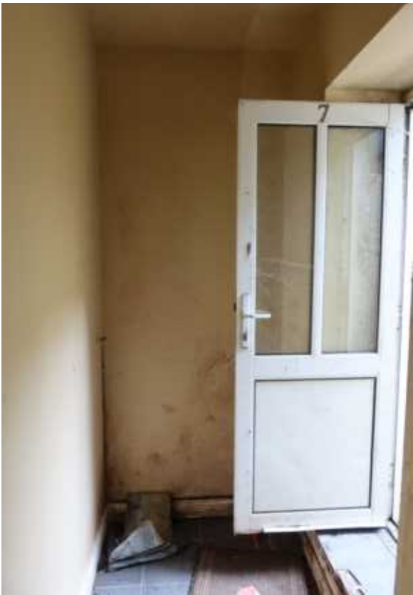
• Fig 33. GF3 entrance.
