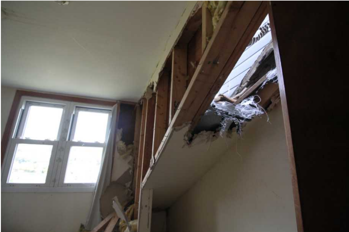
• Fig 102 & 103 Bedroom Top level rear apartment with roof failure.
