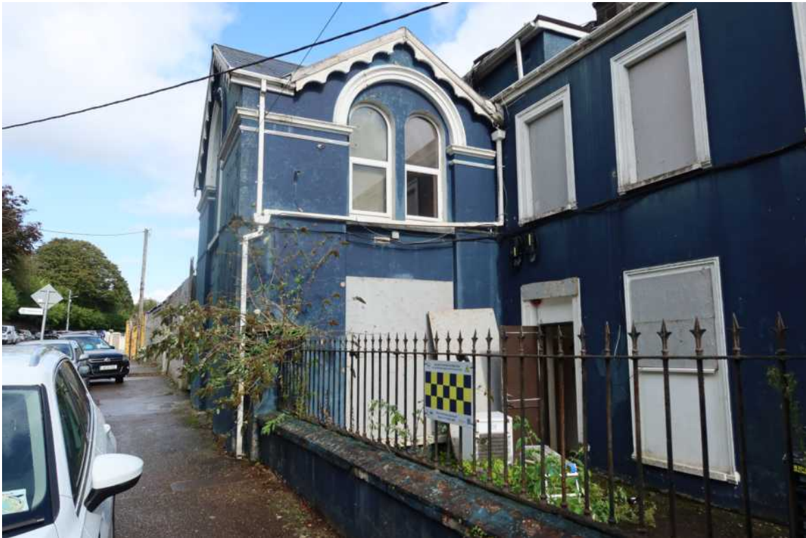
• Fig 22. Wall and railings to South West of house.
