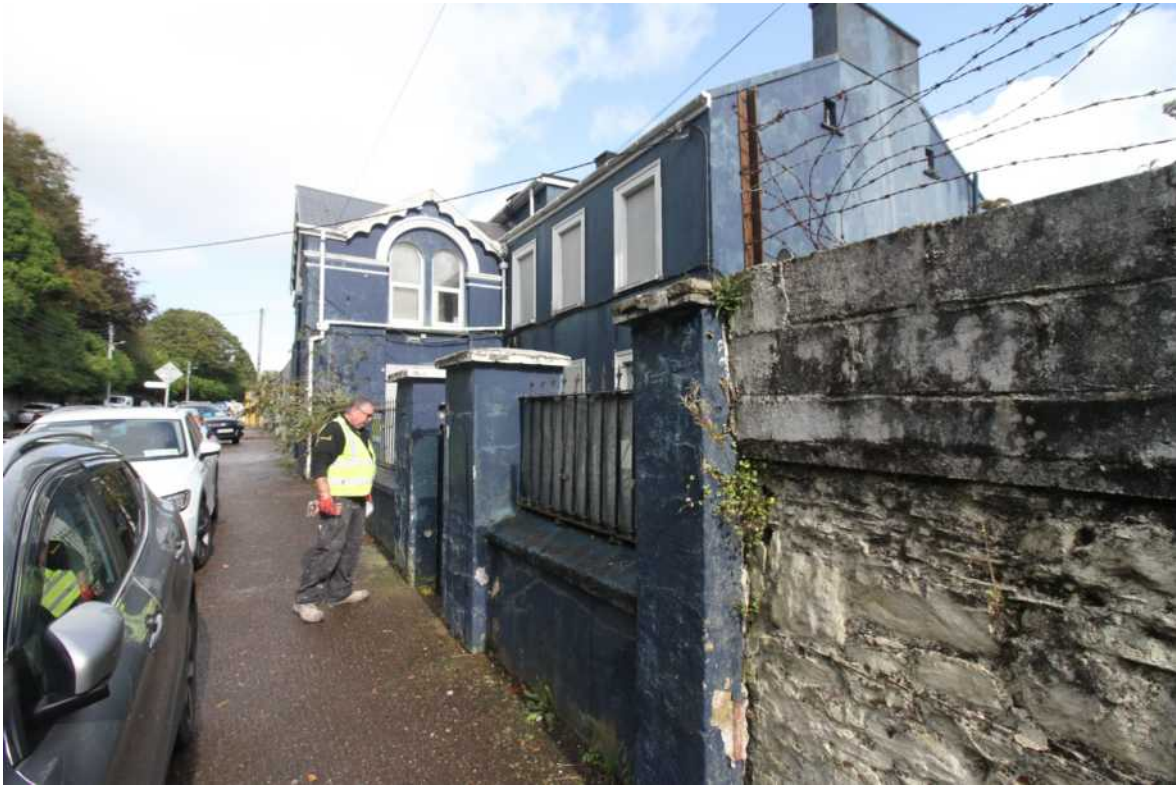
• Fig 23. Wall and railings to South West of house.
