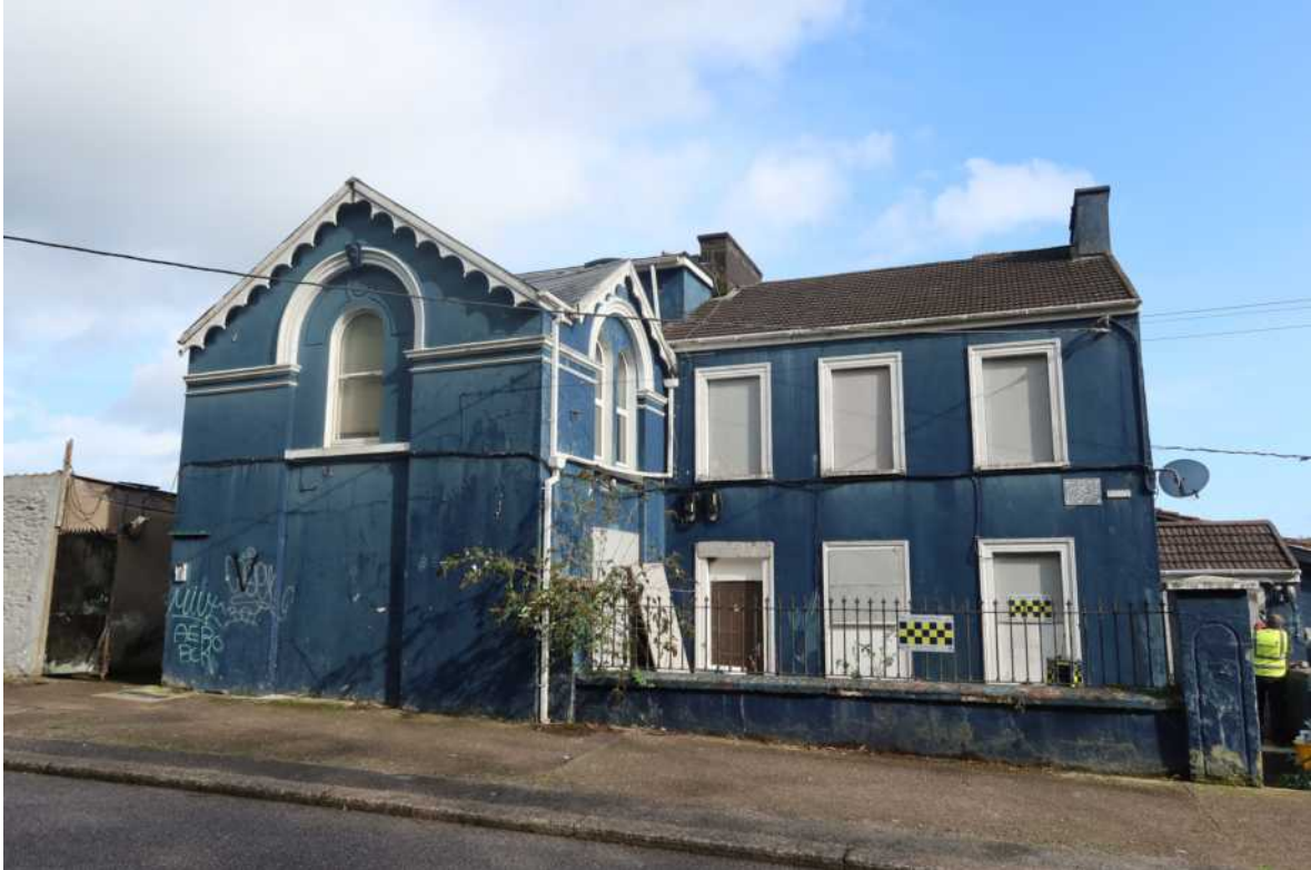
• Fig 9. South West view of house.
