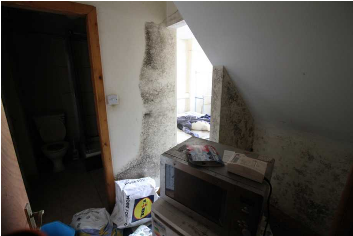
• Fig 100 & 101. Bedroom with common mould issues.
