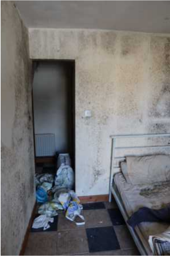
• Fig 89 -92. Typical apartment interiors and damp/ mould issues .
