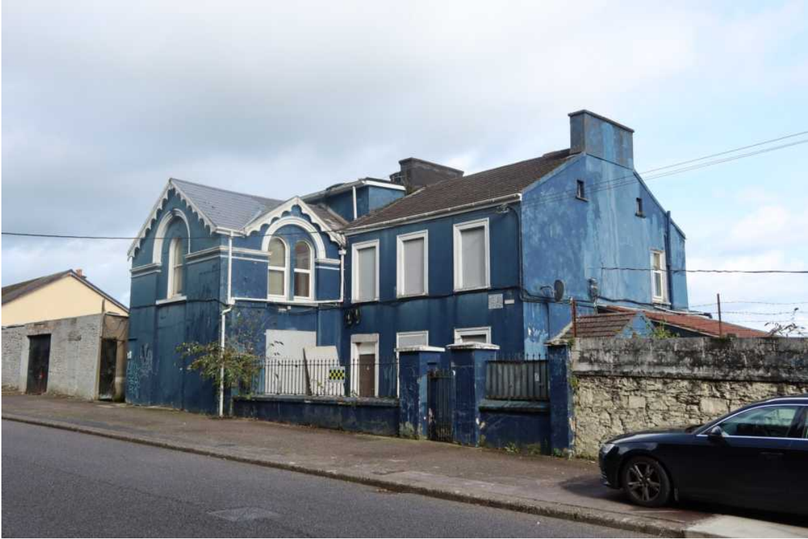
• Fig 11. South West view of house.
