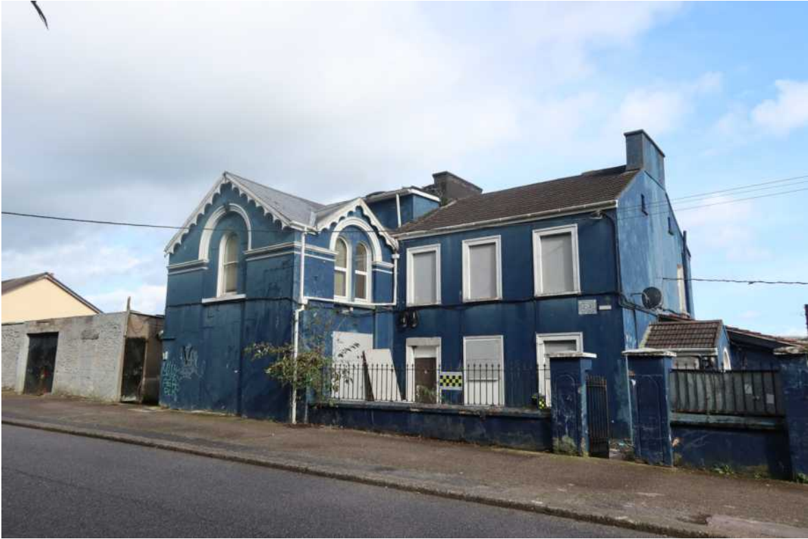
• Fig 10. South West view of house.
