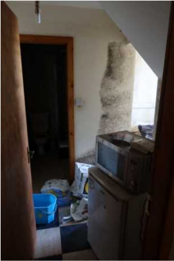
• Fig 89 -92. Typical apartment interiors and damp/ mould issues .
