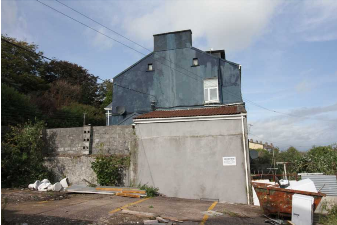
• Fig 12. South end view of house.
