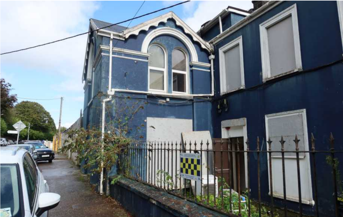
• Fig 34. GF2 entrance, inside railings.
