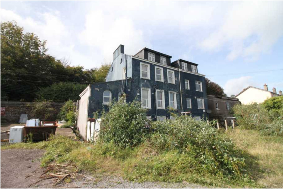
• Fig 15. East South/East view of house.
