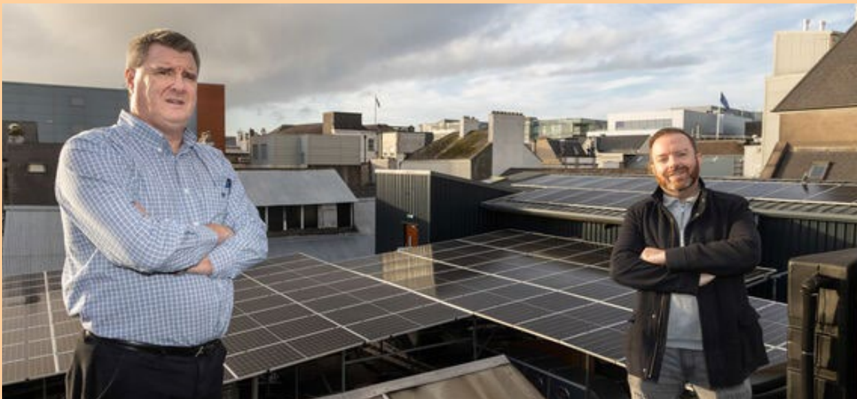
Picture 3 - Solar panels on the rooftop of the Old Oak pub. Kevin Cotteral (L) & Eoin Ahern (R)
