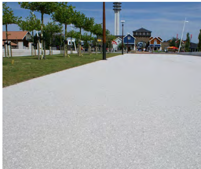
Paving Type 1: Promenade Aesthetic asphalt
