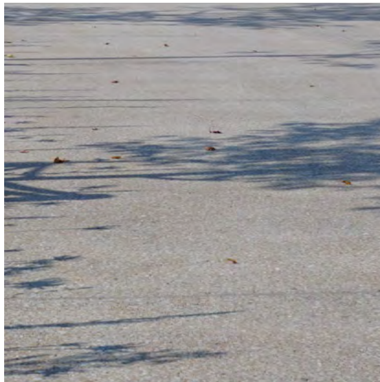
Paving Type 1: Concrete surfaces, mechanically grinded finish
