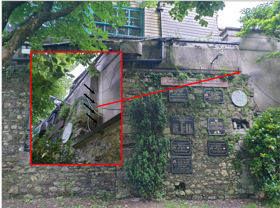
Plate 2. Large vertical crack in wall (inset photograph) at position indicated by arrows
