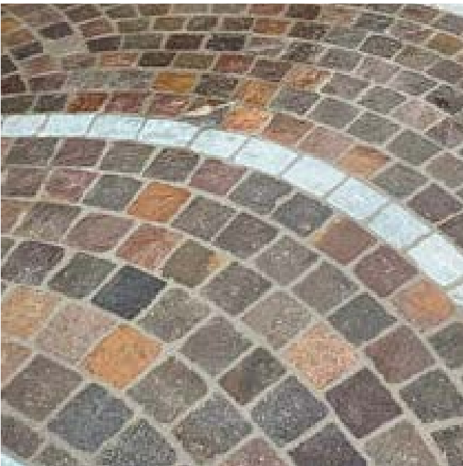
PAVING TYPE E: Three Tone Granite Setts Size: 100 x 100 x 100mm thickness Colour: Mix of reds, brown, greys, and golds
