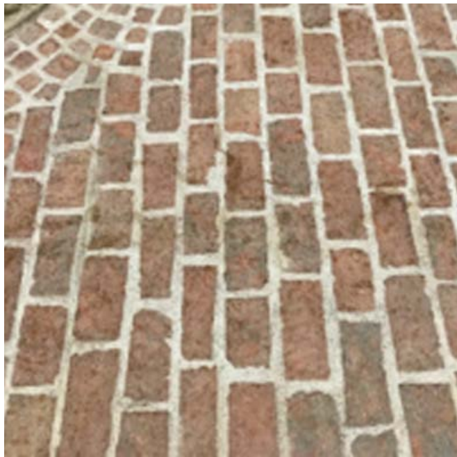
PAVING TYPE D: Granite Paving Setts Size: TBC to match Bishop Lucey Park Colour: Red Granite
