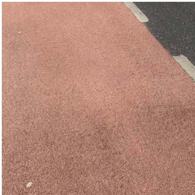
PAVING TYPE G: Red Chip Asphalt at Cycle Lane Size: To Engineers Details Colour: Red
