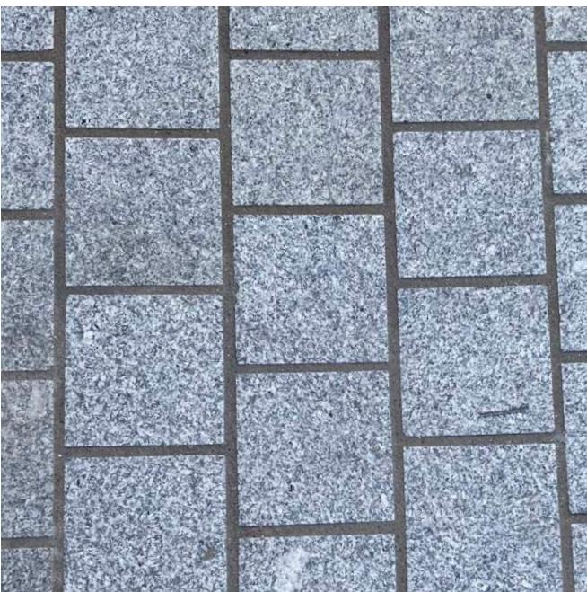
PAVING TYPE B: Granite Paving Setts Size: 150 x 150 x 150mm thickness 150 x 150 x 100mm at building threshold Colour: Light Granite (G-B-010)
