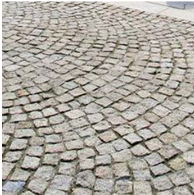
PAVING TYPE C: Granite Block Paving Size: 100 x 100 x 100 mm limestone cobbles, fan-tail pattern Top of Hill: Varied 100-150mm x random lengths Colour: Blue Grey
