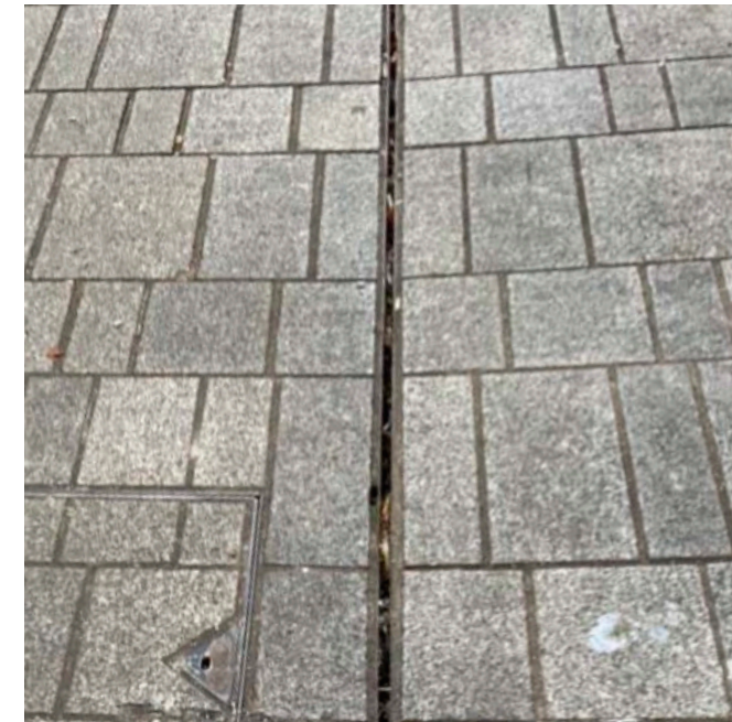
Slot Drain seamlessly integrated into paving
