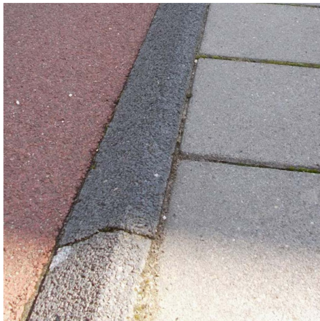
KERB TYPE 3: Chamfered Stone Kerb at Cycle Lane
