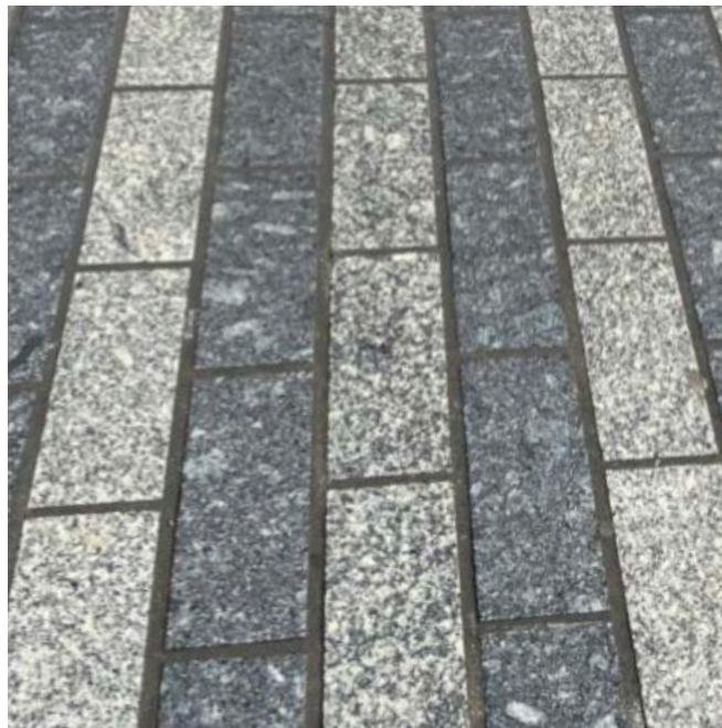
PAVING TYPE F: Granite Block Setts (alternating pattern) Sizes: 100mm thickness Colour: Light Granite and Dark Granite
