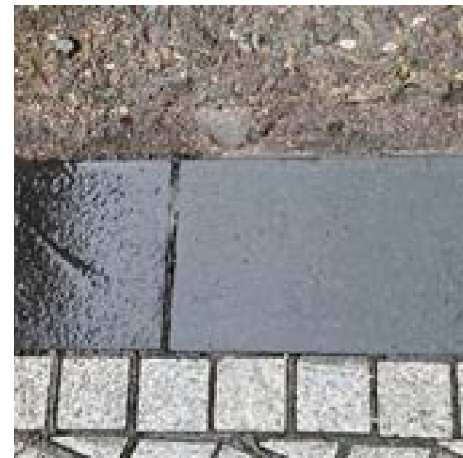
KERB TYPE 2: Flush Kerb (Stone Banding)
