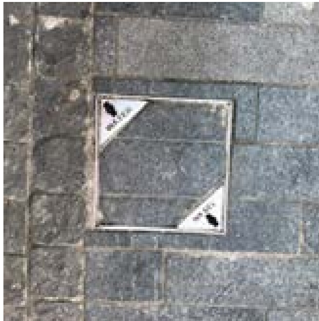
Galvanized recessed manhole covers where required
