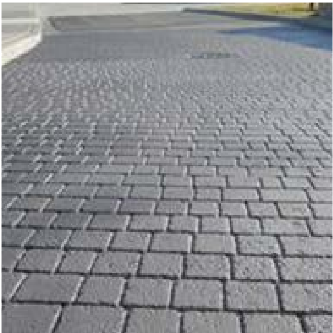
PAVING TYPE B: Street Print Asphalt Size: To Engineers Details Colour: Dark Grey
