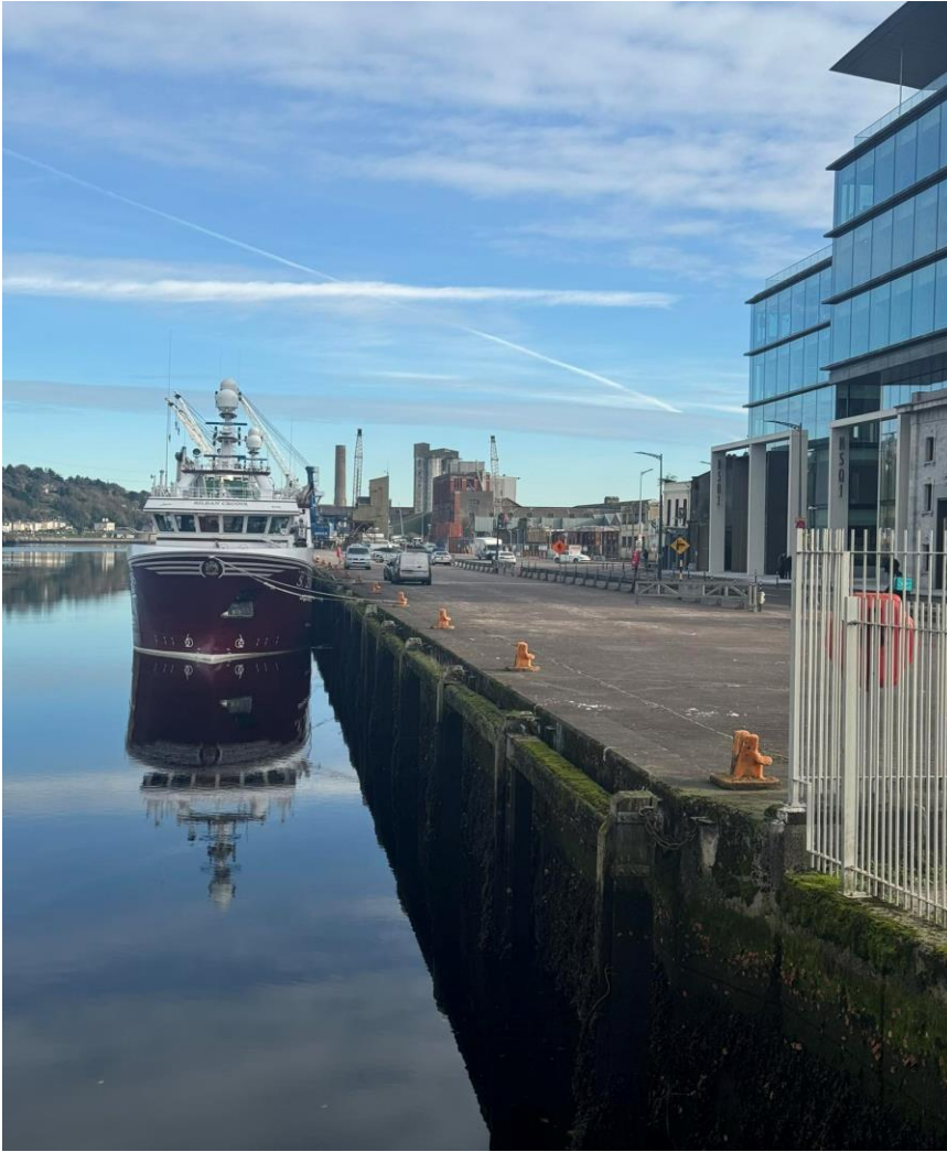
Photograph 2: Existing wharf on Albert Quay East looking downstream. The existing RC quay wall is fronted by steel sheet piles with intermittent timber fenders.
