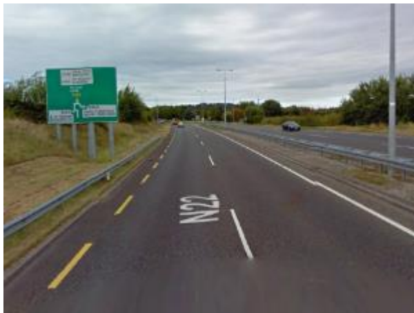
Figure 3.8: Ballincollig Bypass (N22)
