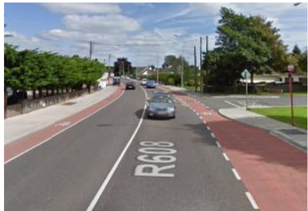
Figure 3.5: R608 (public road access on right)
